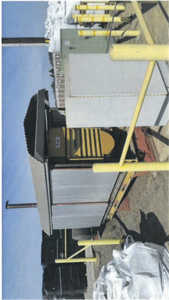
Backup generator w/ 200 gallon diesel tank
