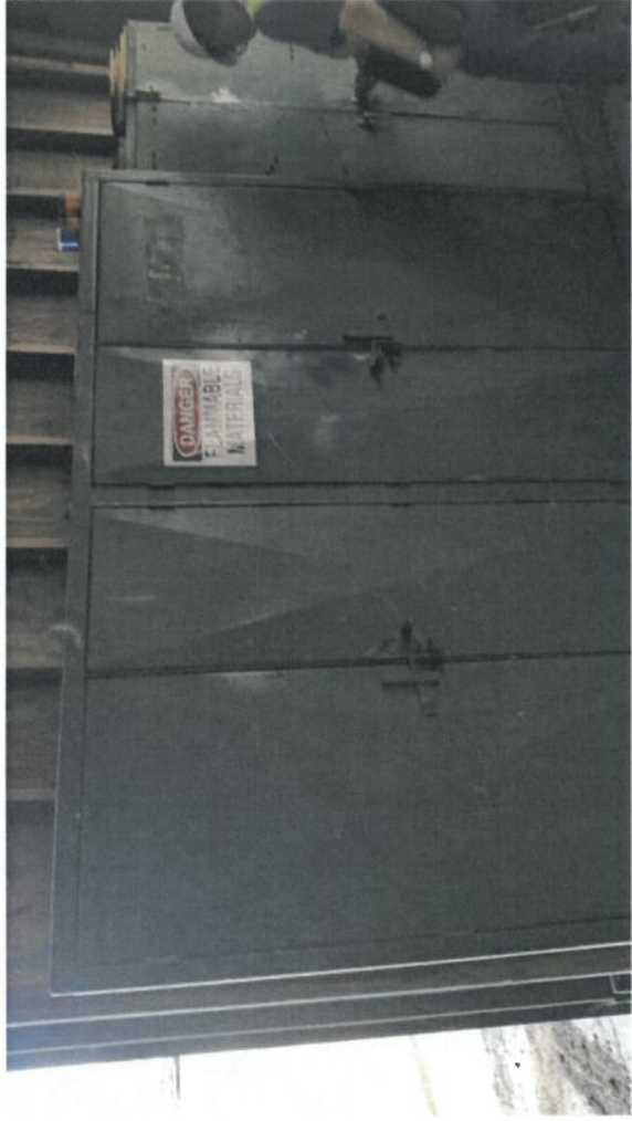
Metal Storage lockers for household sized hazardous materials (paint, varnish, solvents, glues)
