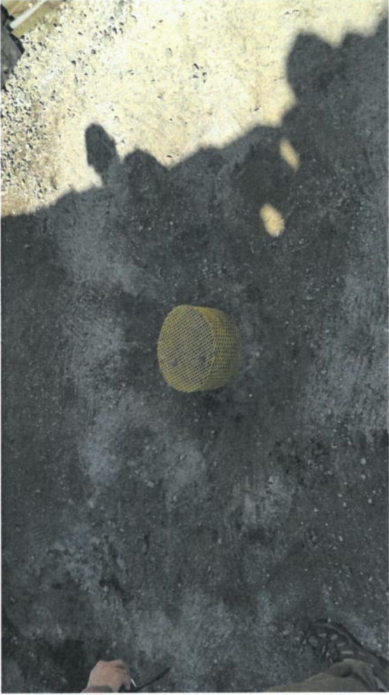
Exterior Drain - between building 4 and 5
