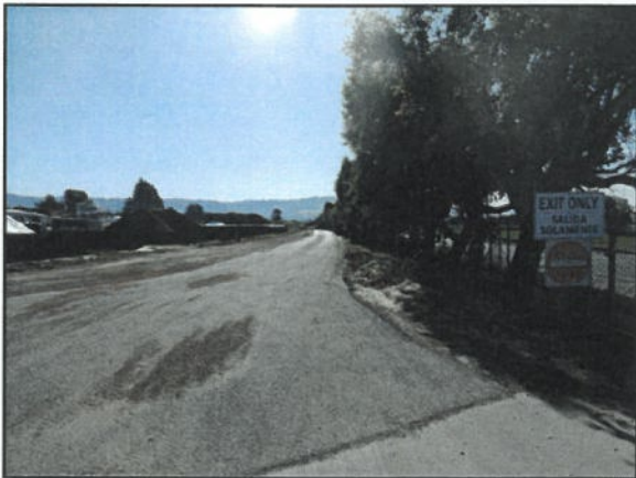
Photograph 3. Access road (facing east).
