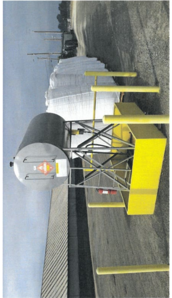
500 gallon Gasoline AST w/ Secondary Containment
