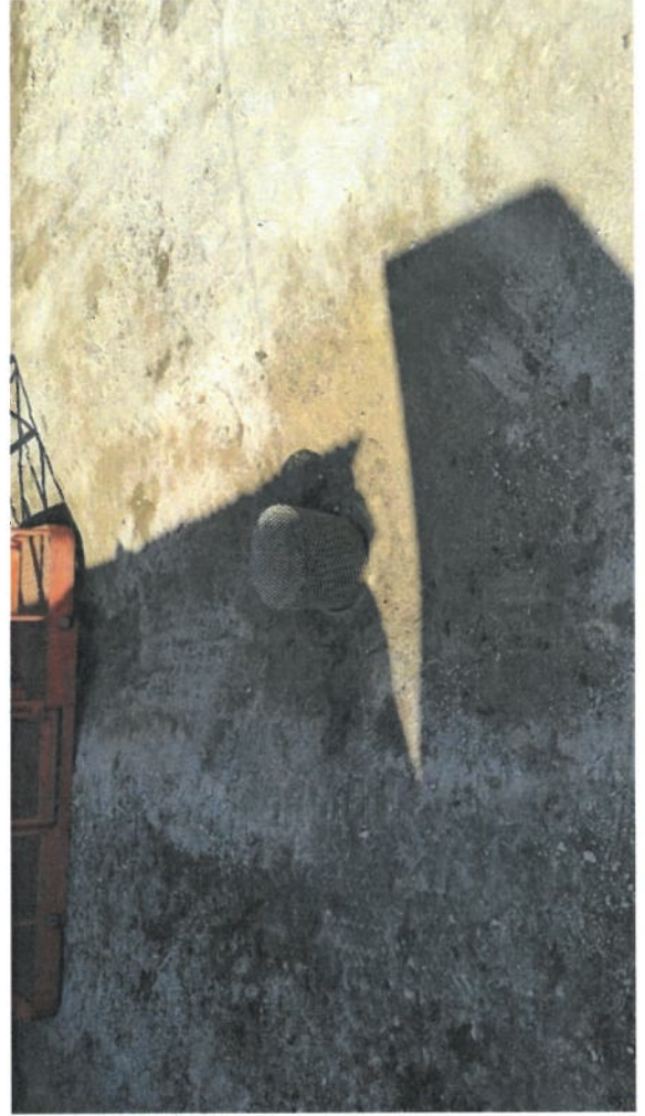
Exterior drain - between building 5 and 6
